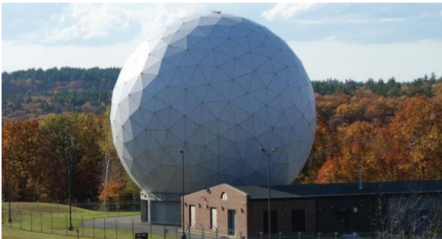
Remote Tracking Station
